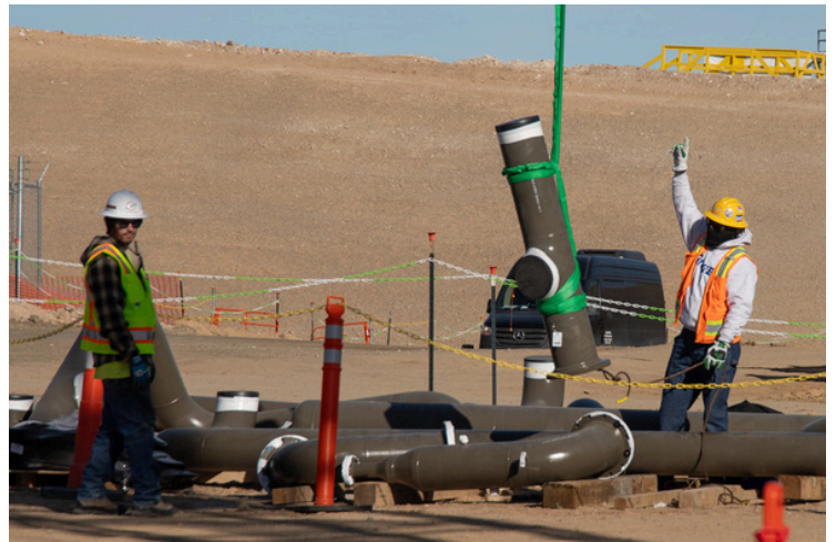
The first aboveground pipe installed: a 288-pound carbon steel section was craned into the Filter Building in late January 2026.
