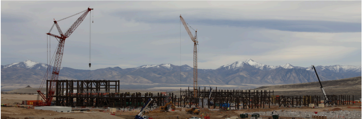
Structural steel advanced at the Filter Building, Magnesium Sulfate Building and Liquid Sulfur Tanks.
