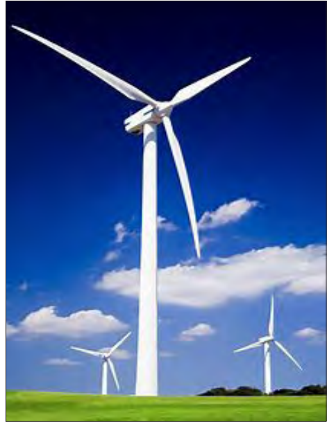
A wind turbine may contain 335 tons of steel, 4.7 tons of copper, 13 tons of fiberglass, 3 tons of aluminum and 1,200 tons of reinforced concrete.
